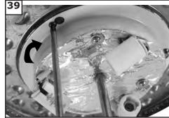
Place light kit over 3 screws and twist in direction of arrow to hold in place. Then tighten all 3 screws securely.
